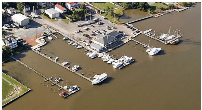
An overhead view of Chestertown Marina. The Town of Chestertown owns the four piers to the right, while the lower dock is private property.
