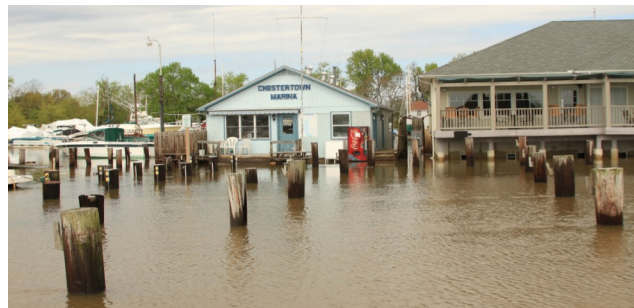
High tides cause flooding throughout the Marina site.
