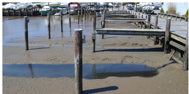
Low winter tides reveal excessive siltation and the need for dredging.
