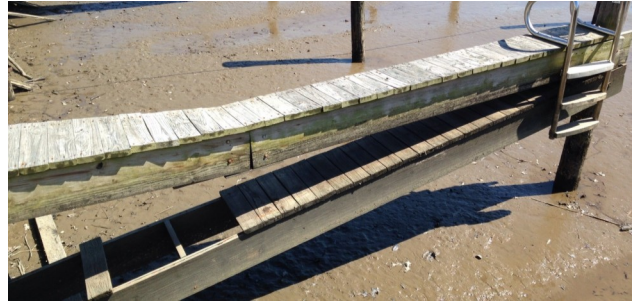
An old dock that has collapsed and needs to be replaced.
