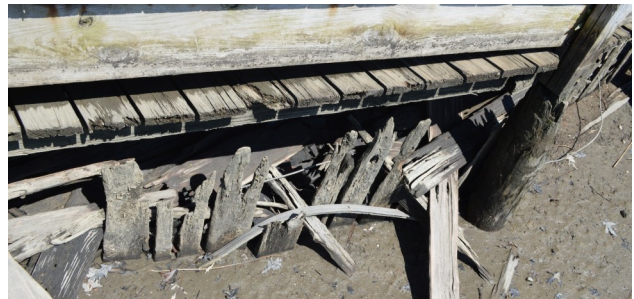
The current state of the bulkheads at Chestertown Marina.
